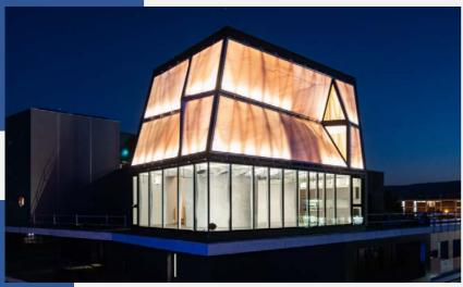
Completed DFAB HOUSE, featuring a lightweight translucent façade with thermal insulation properties (Copyright Roman Keller / NCCR Digital Fabrication)
